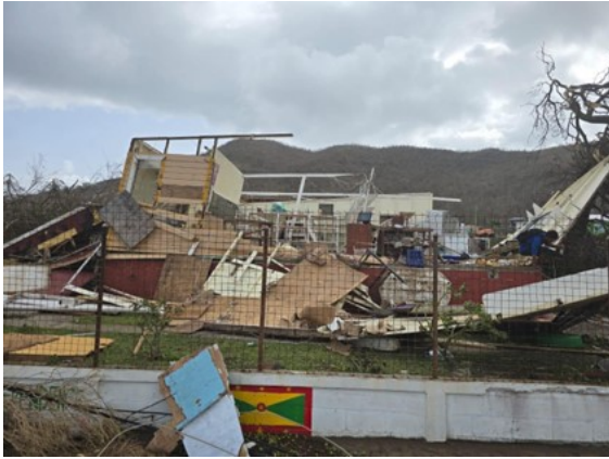
Figure 2: Assessing damage from Hurricane Beryl on July 3, 2024
